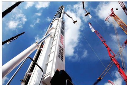
Construction Site And Light Industry
